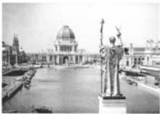
Looking West From the Peristyle
